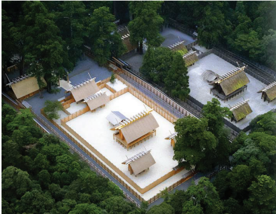
Figure 1. Ise Jungu, new shrine construction adjacent to old shrine 9
